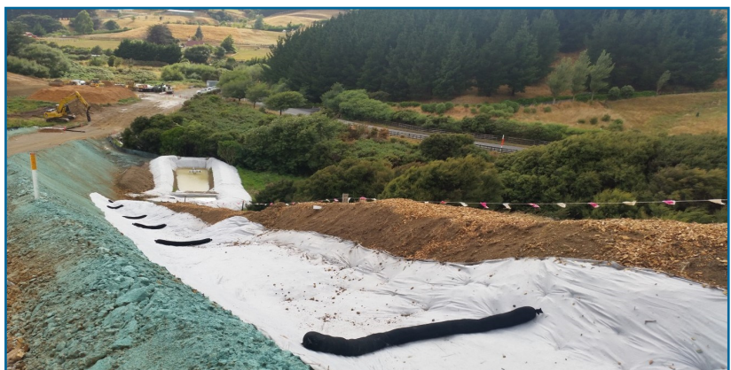
Sediment Retention Pond at the Bradey Track (Bradey Road in the background)
