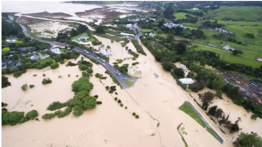
The Pāuatahanui Roundabout 15 November 2016 (Jack Scott, NZ Drones Ltd)
