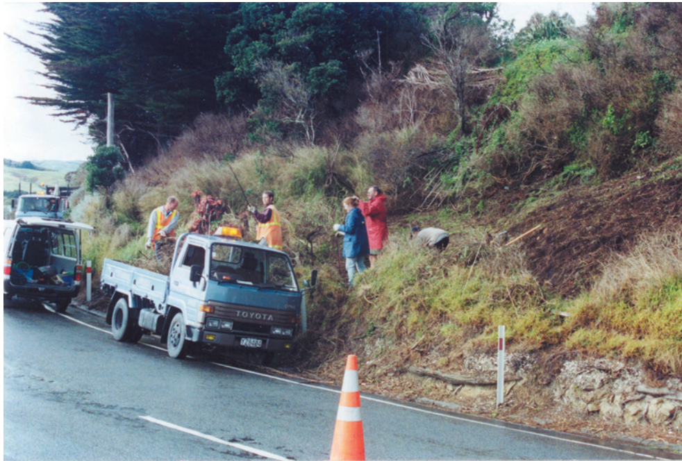
Figure 3. Clearance of Site R27/24 in preparation for excavation.
