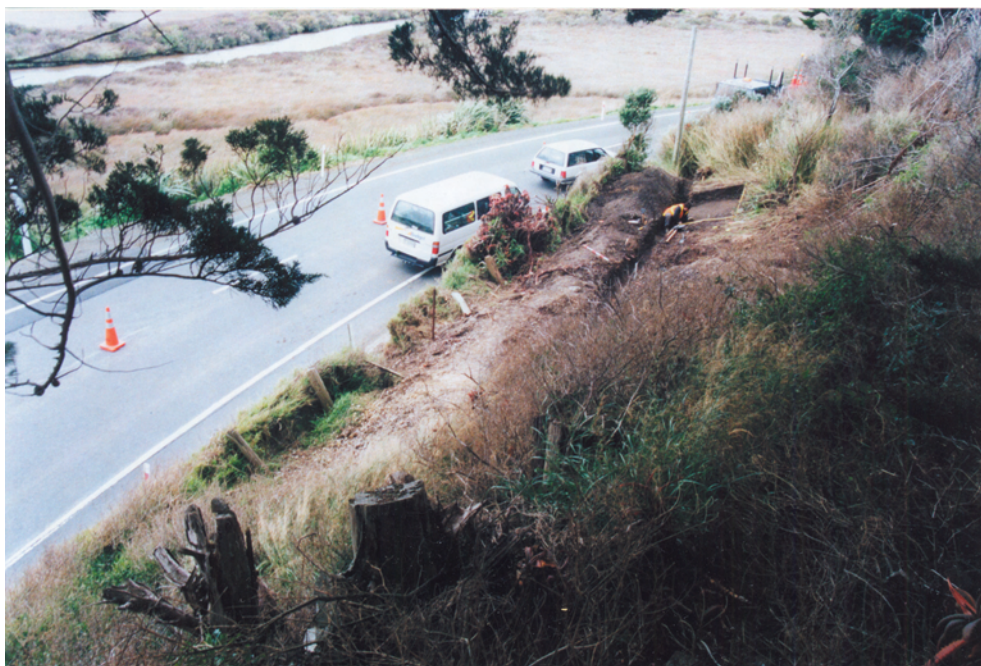
Figure 4. Excavation in progress, looking east towards Area D.
